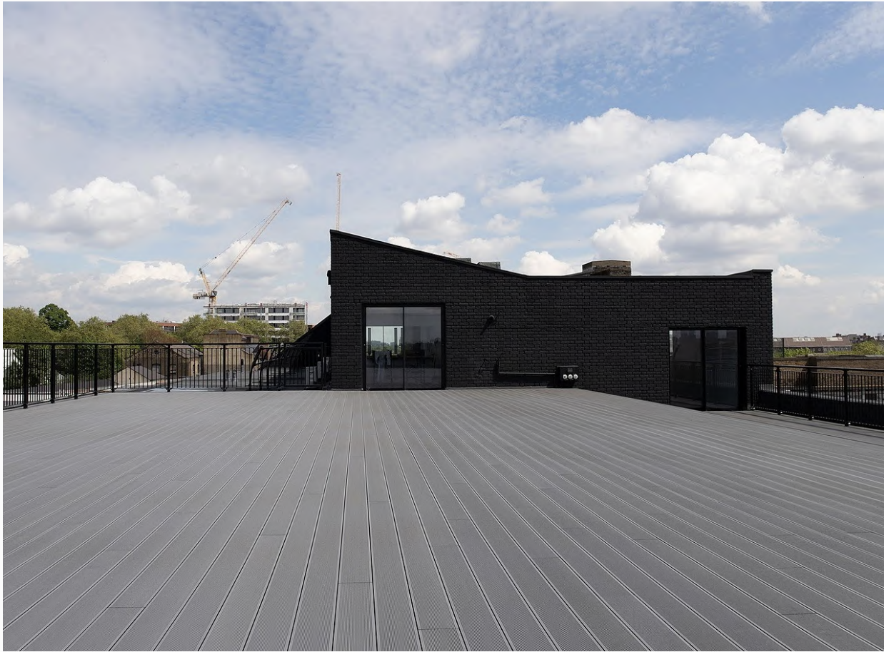
Overview of roof
